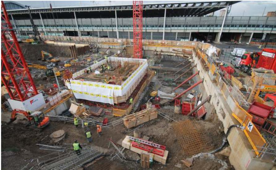
*Slipform core formwork completion and right, forming basement pool slabs around props*
