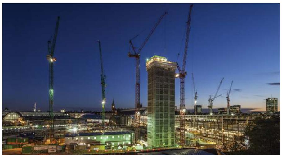
*©John Sturrock & Argent – 24 hour slipforming operations, a first for Argent at King's Cross*
